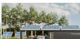
Stand alone Off Grid Solar System
